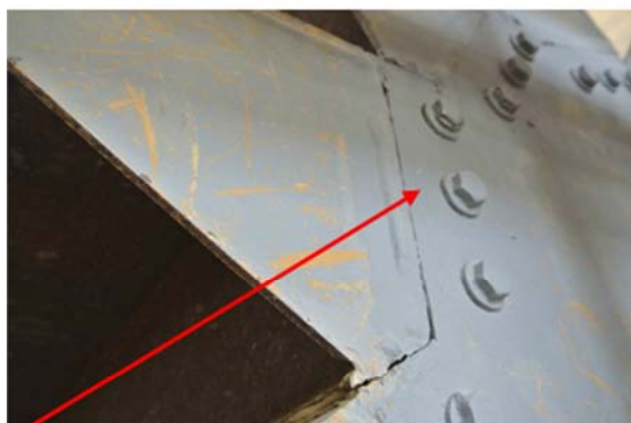
loosened bolts at the turbine blades
