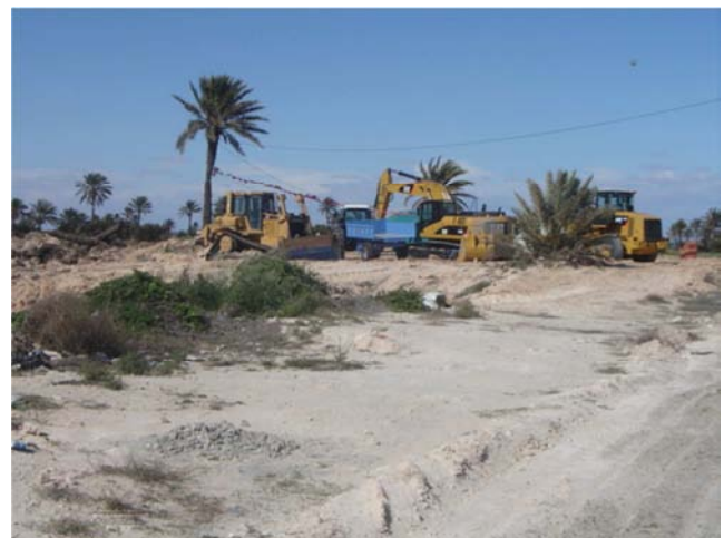
Figure 10. Bulldozers tearing palm trees, 2007.
